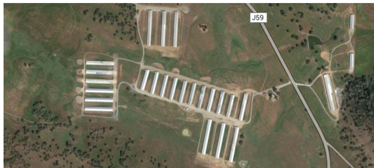
Figure 8 - Google maps view of the barns at Diestel's Jamestown facility visited by investigators.
